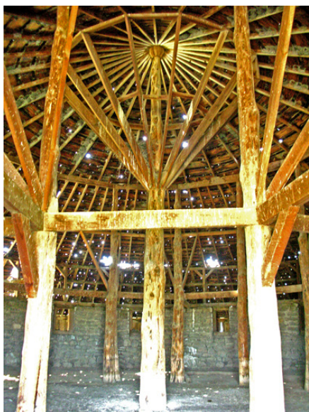
Malheur, Oregon Structural Beams in a Round Barn used for Exercising Horses in Winter
