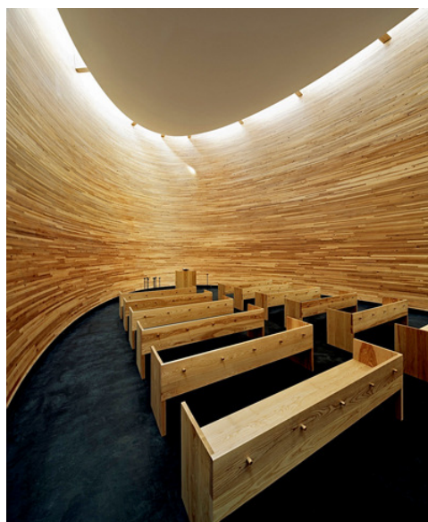
Helsinki, Finland Kamppi Chapel, fabricated via CAD design and Glulam construction using smaller 3 rd Growth Trees
