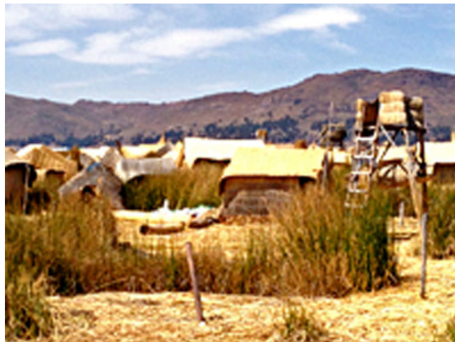
Lake Titicaca, Peru Floating Islands and Structures made from Bundling Water Reeds
